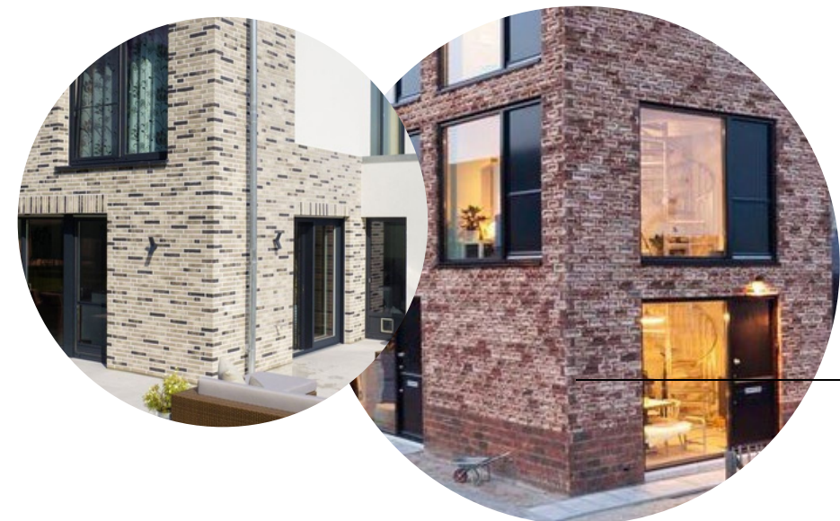
Thin bricks - Lightweight brick facade Feldhaus klinker - Thin bricks
